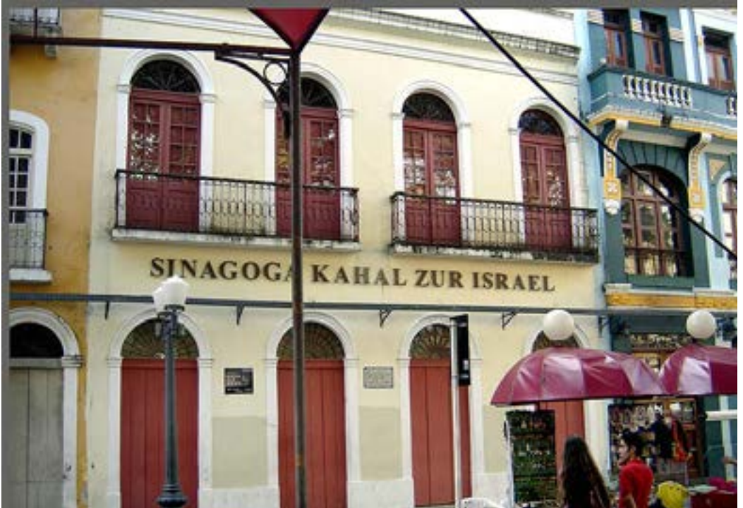
Exterior view of the synagogue
